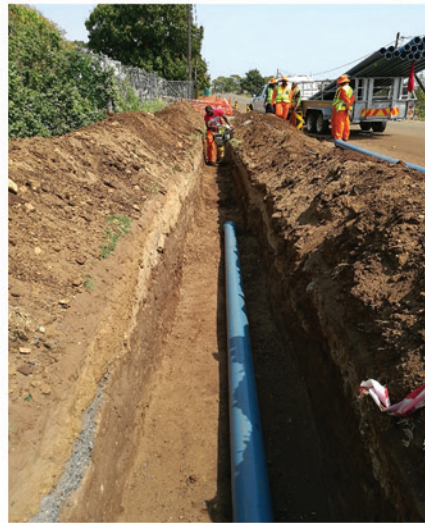
eNseleni Trench Compaction before laying pipe
