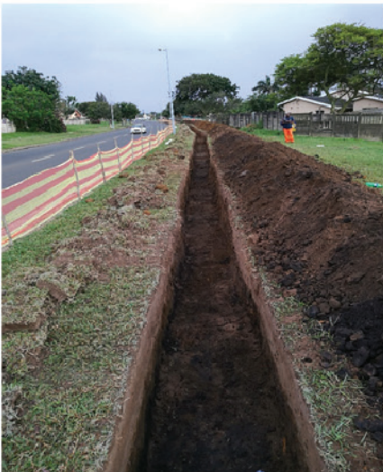
Richards Bay Trench Excavation
